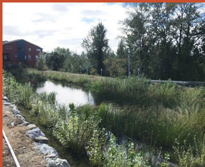
Stormwater pond at Greenbridge
